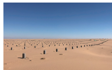
▲ Supporting pile foundation laid out
